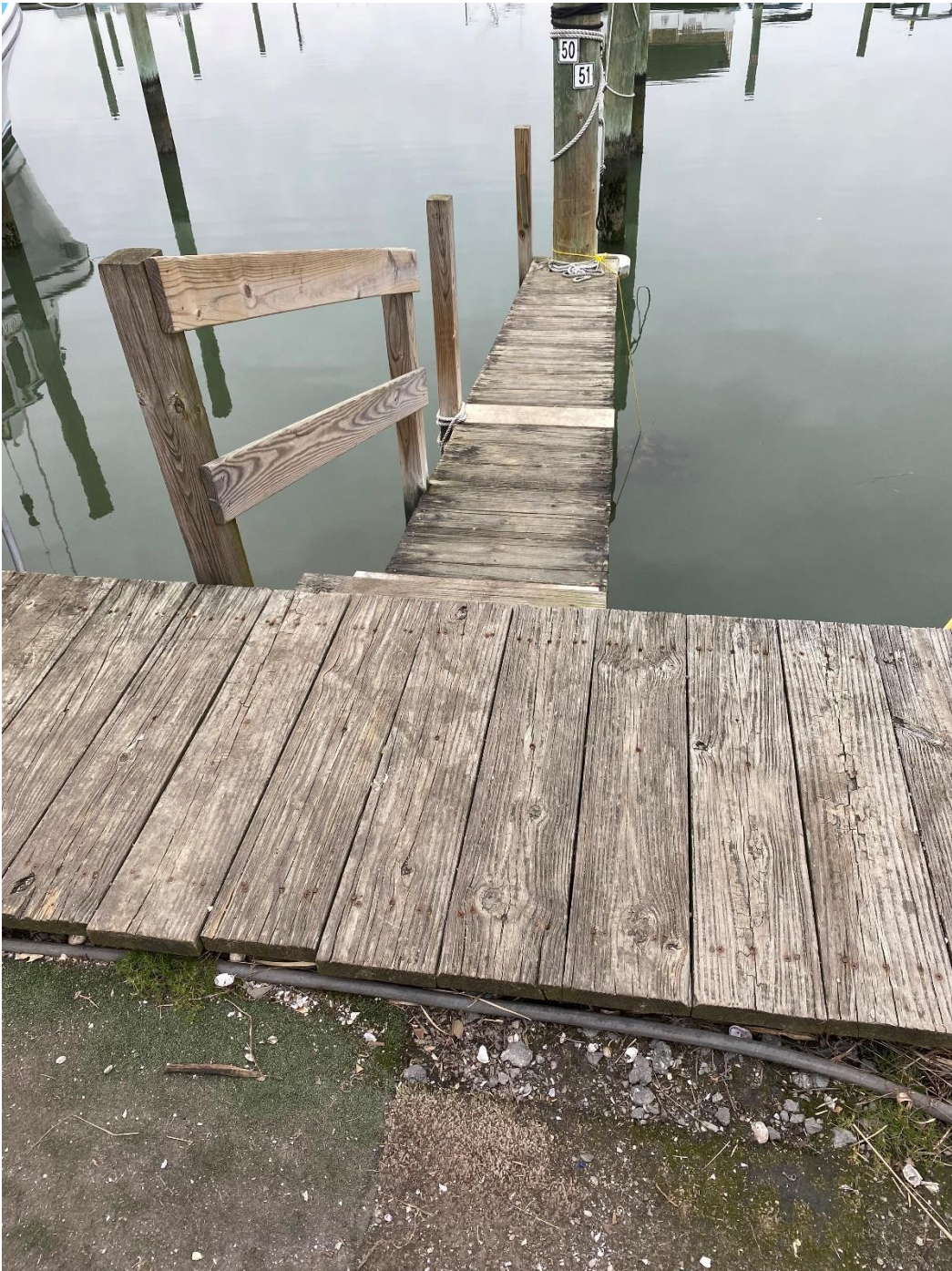
Replacing Finger Piers at Harbor.
